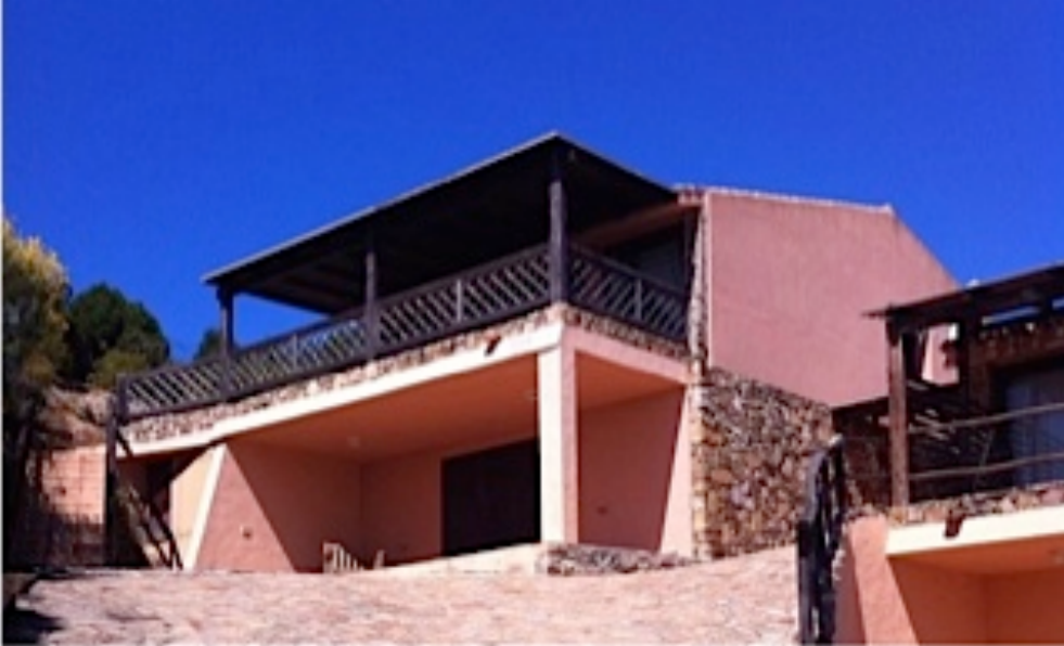
south facade before
